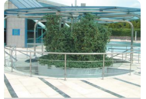
KANOPI İSTANBUL BORSA CANOPY İSTANBUL EXCHANGE
