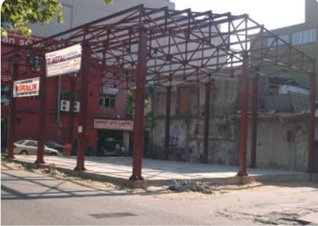
SEYRANTEPE / ÇELİK BİNA / 25 TON SEYRANTEPE / STEEL BUILDING 25 TONS
